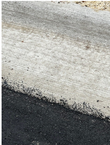
Asphalt against Curb and Gutter
